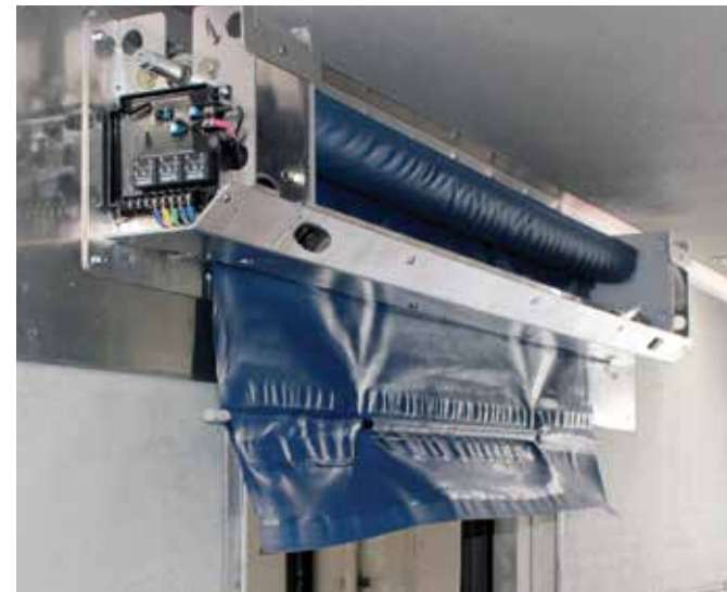
A side-door electric unit being installed in Florida. The unit is missing the tracks where the blue barrier runs up and down.
